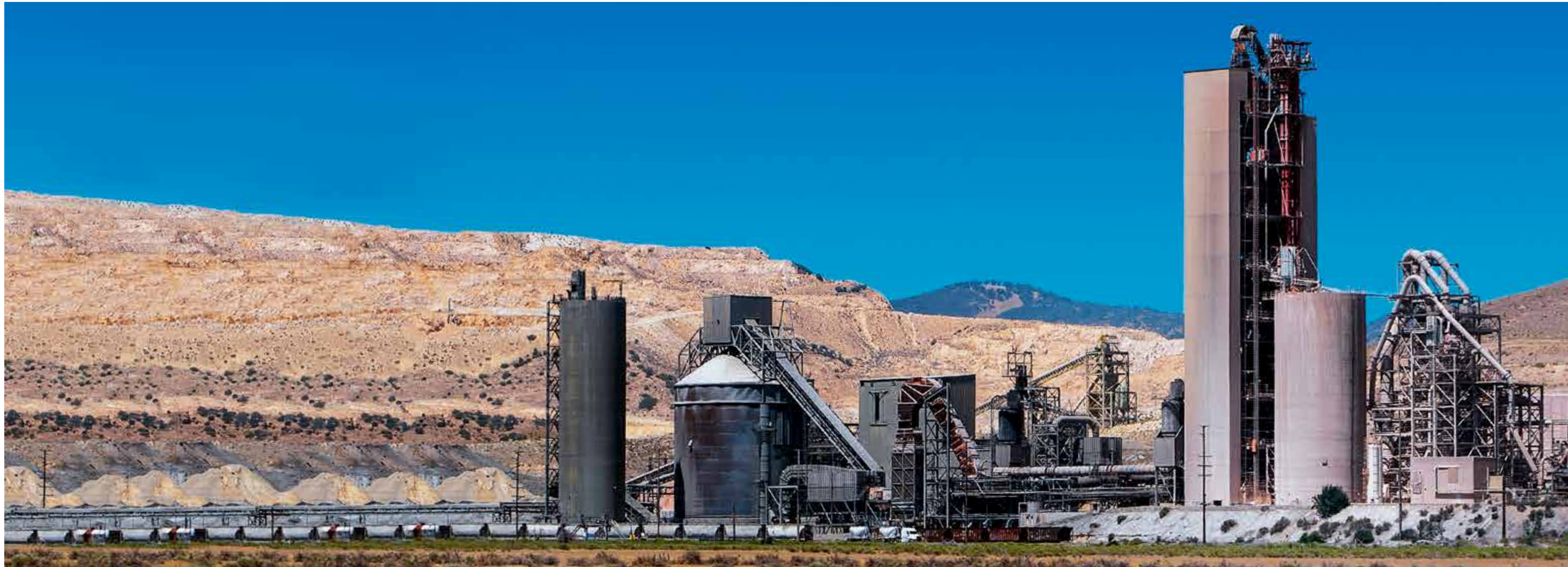
Tehachapi Cement. Tehachapi, California, EE.UU.
