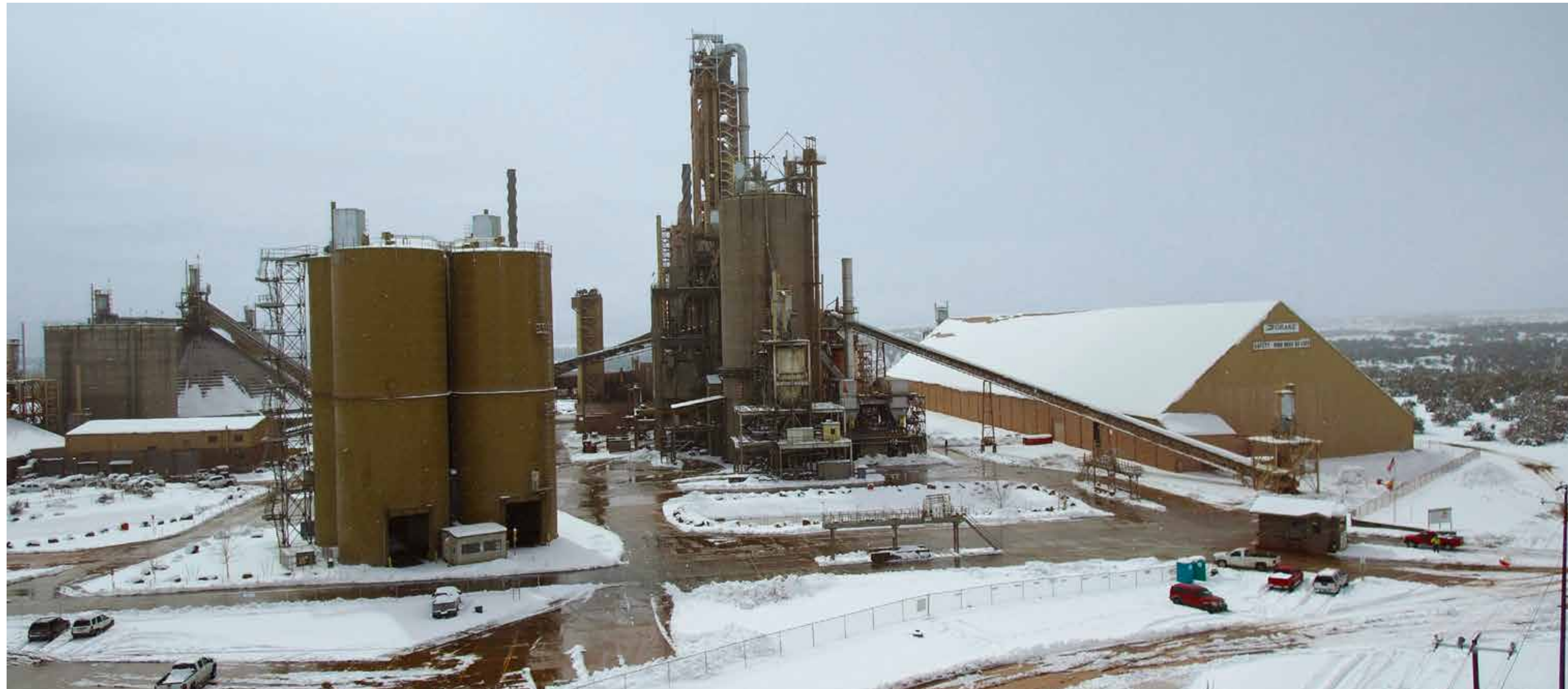
Drake Cement. Arizona, EE.UU.
