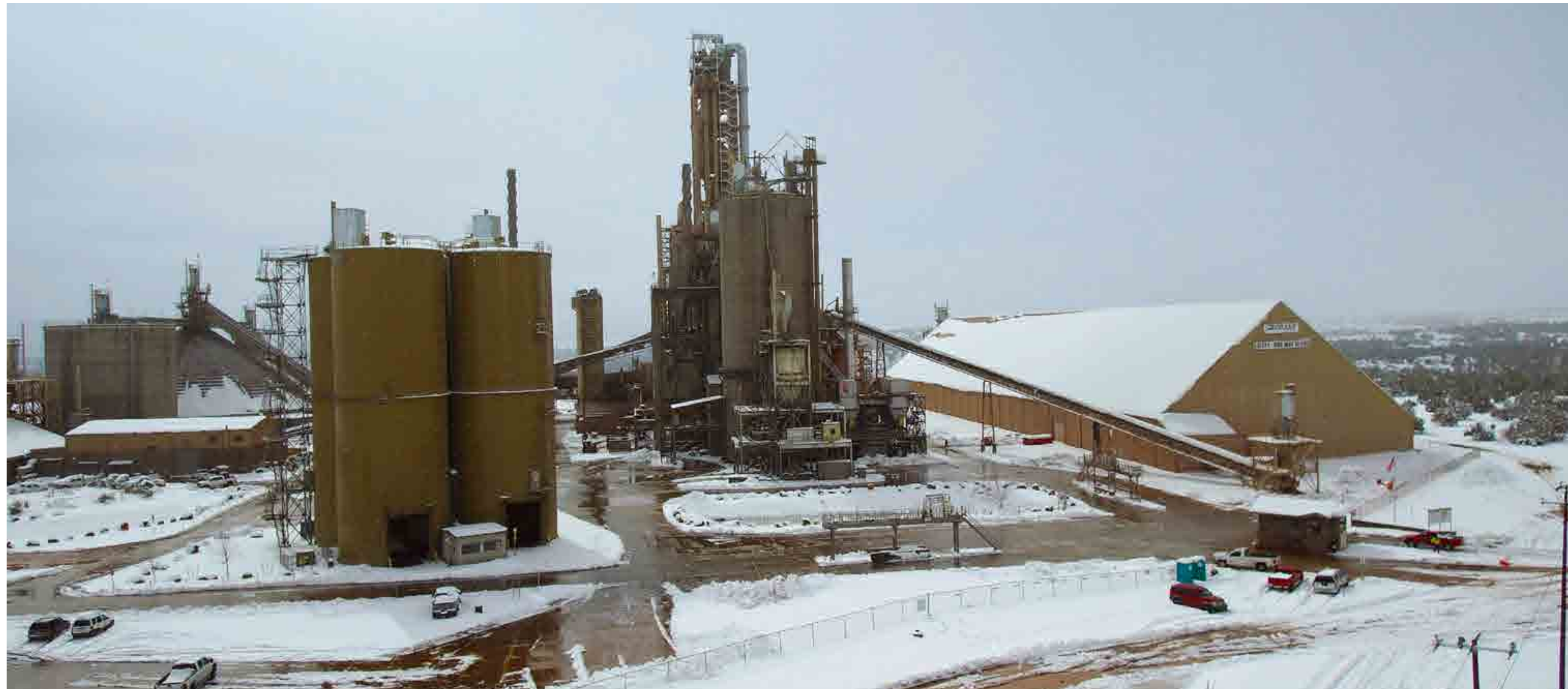
Drake Cement. Arizona, EE.UU.
